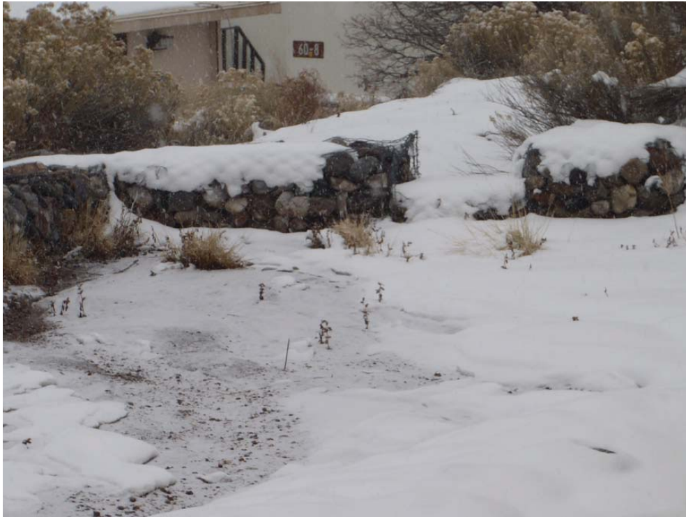
Rock gabions to channel storm water flow and prevent erosion
