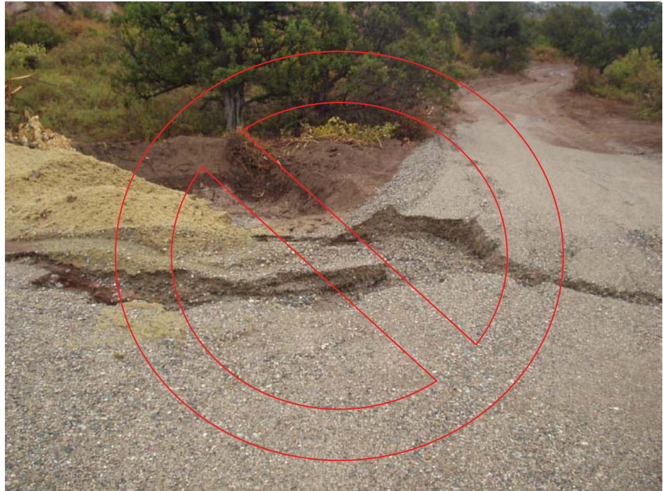
Base course should not be used for stabilization in areas of high flow.
