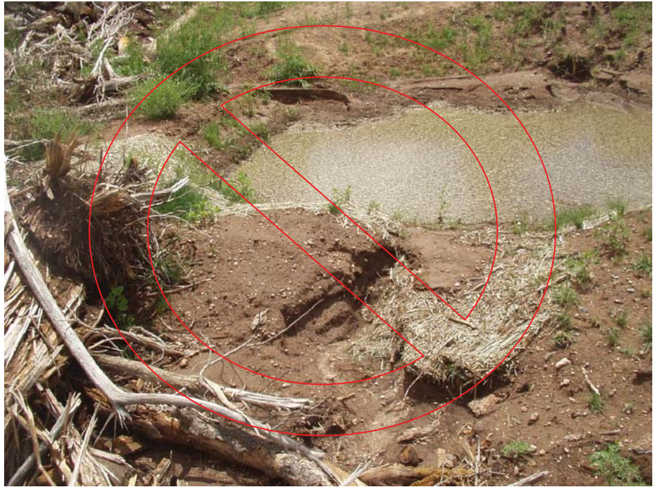
There is no defined/armored pathway for water to flow in and out of the pond.
