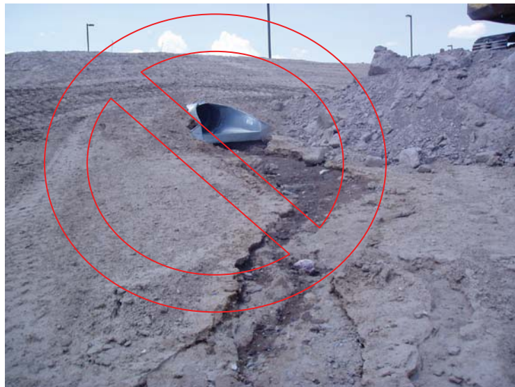
Properly installed riprap at culvert outlet will control erosion.
