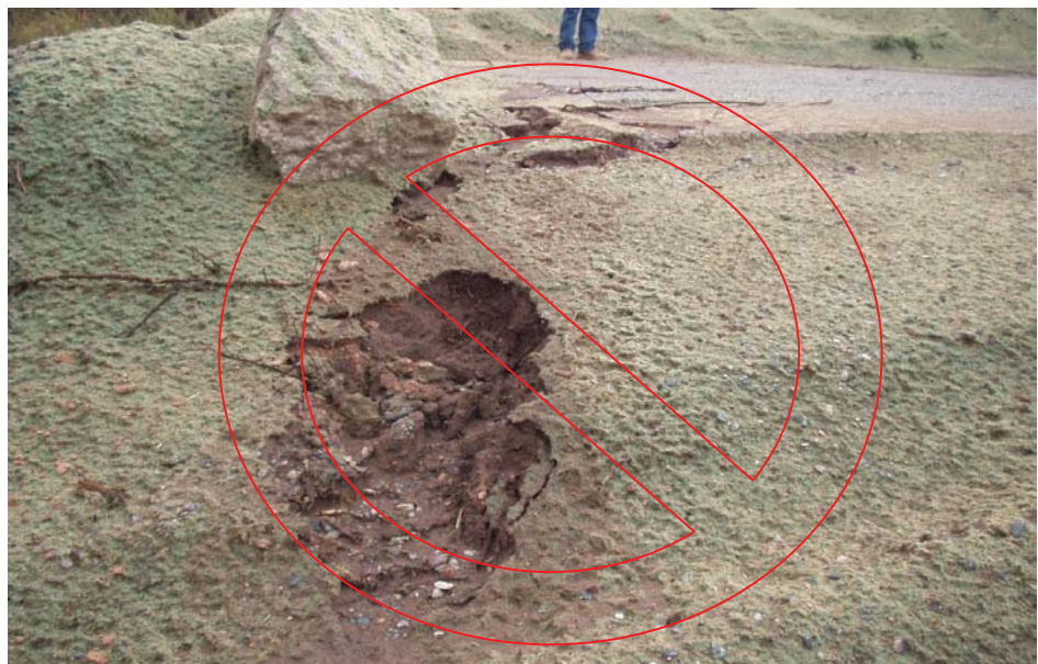
Hydromulch should not be applied too lightly or in areas of high flow.
