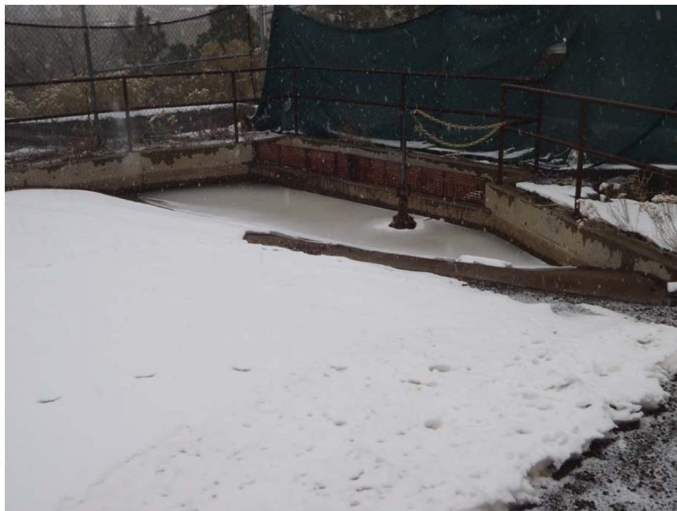
Pond to capture storm water and settle out solids
