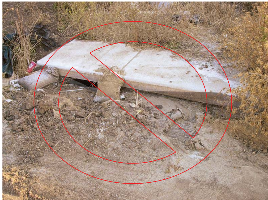
Remove sediment and debris in a timely manner from storm drains.
