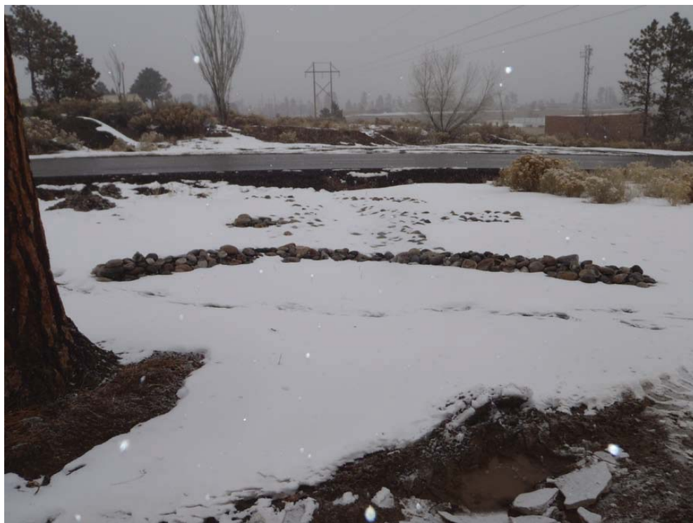
Rock rundown and berm to channel storm water flow
