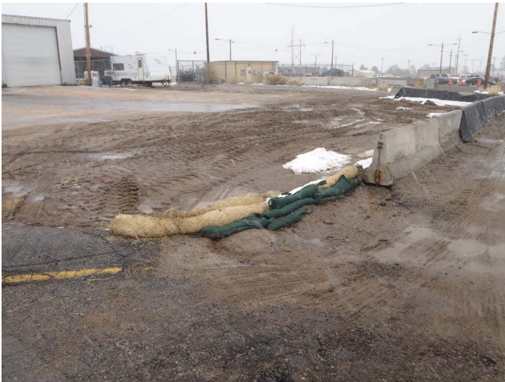
Straw wattles and gravel bags to prevent sediment transport
