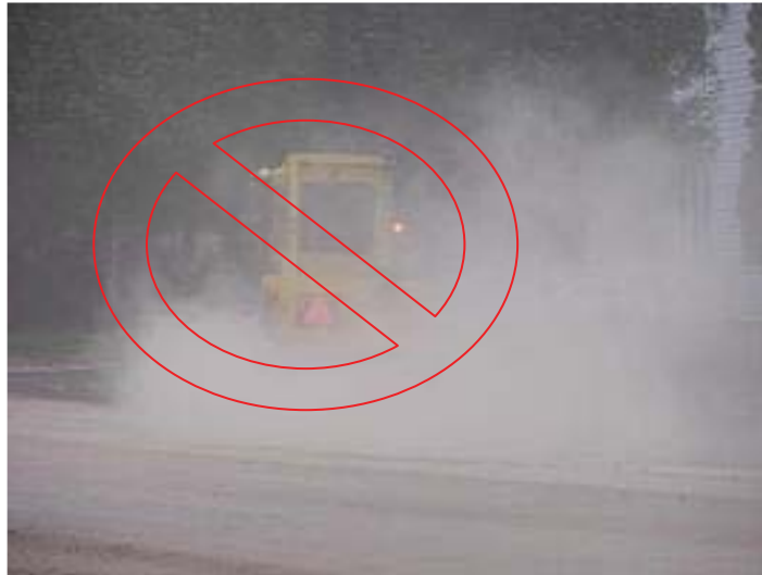
Sweeping without vacuuming causes severe dust migration leading to sediment transport offsite.
