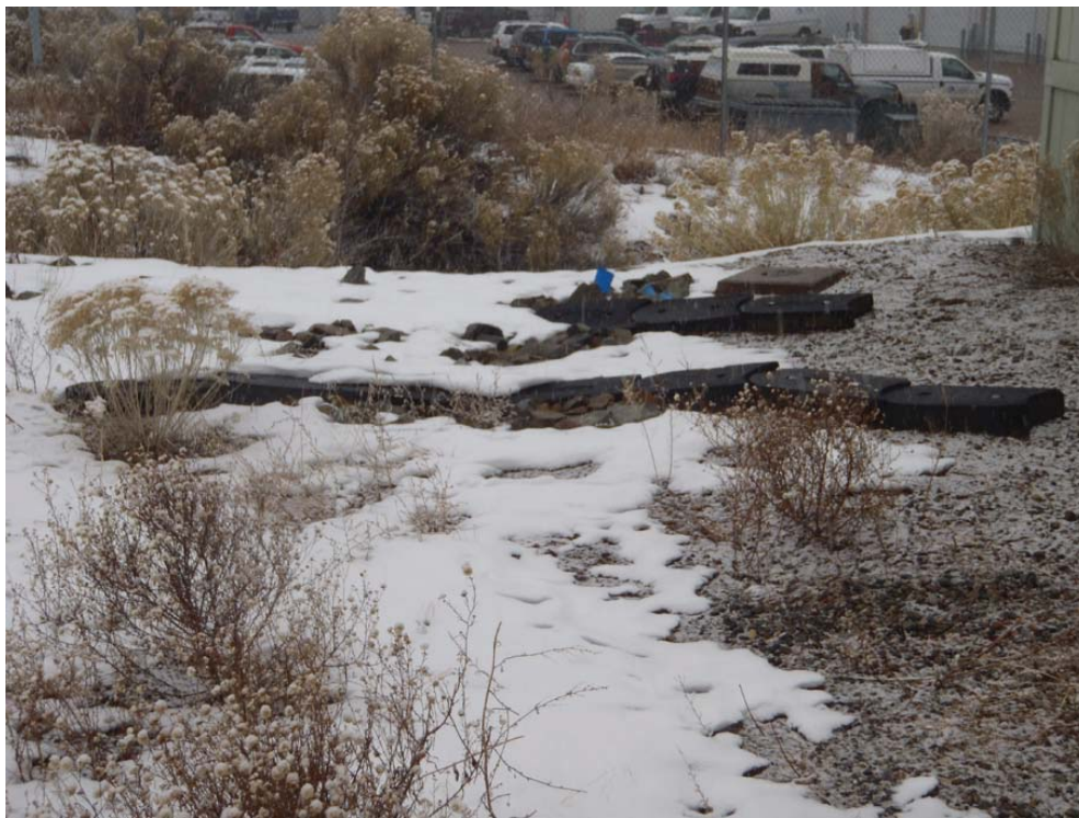
Eco-Block and a rock run-down
