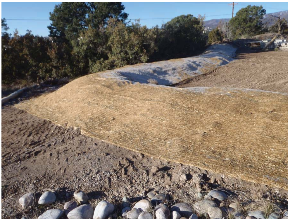
Matting to stabilize a disturbed area and prevent erosion
