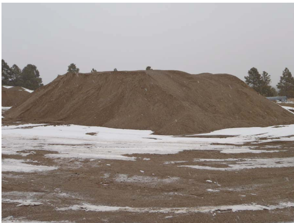
Sediment can be transported with storm water from material piles like this without controls
