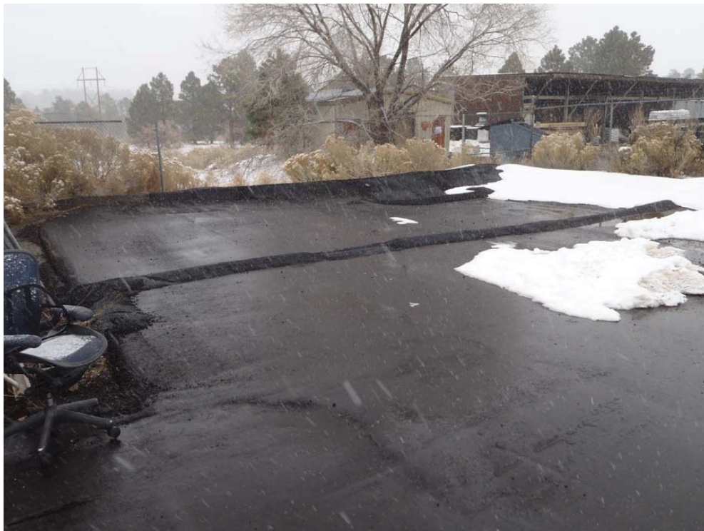
Storm water drainage culvert and asphalt berms
