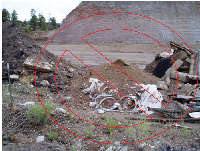
Improper waste disposal and storage of waste products. Containerize and separate waste items for proper disposal.
