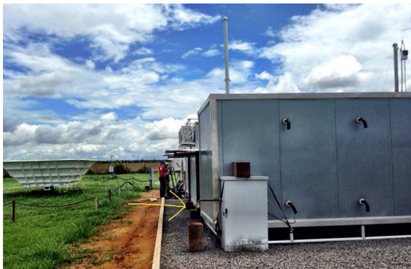
Figure 1. Photograph from the T3 field site. The NAIS instrument is inside the white box next to the container. The yellow arrow points to the NAIS inlet tube.
