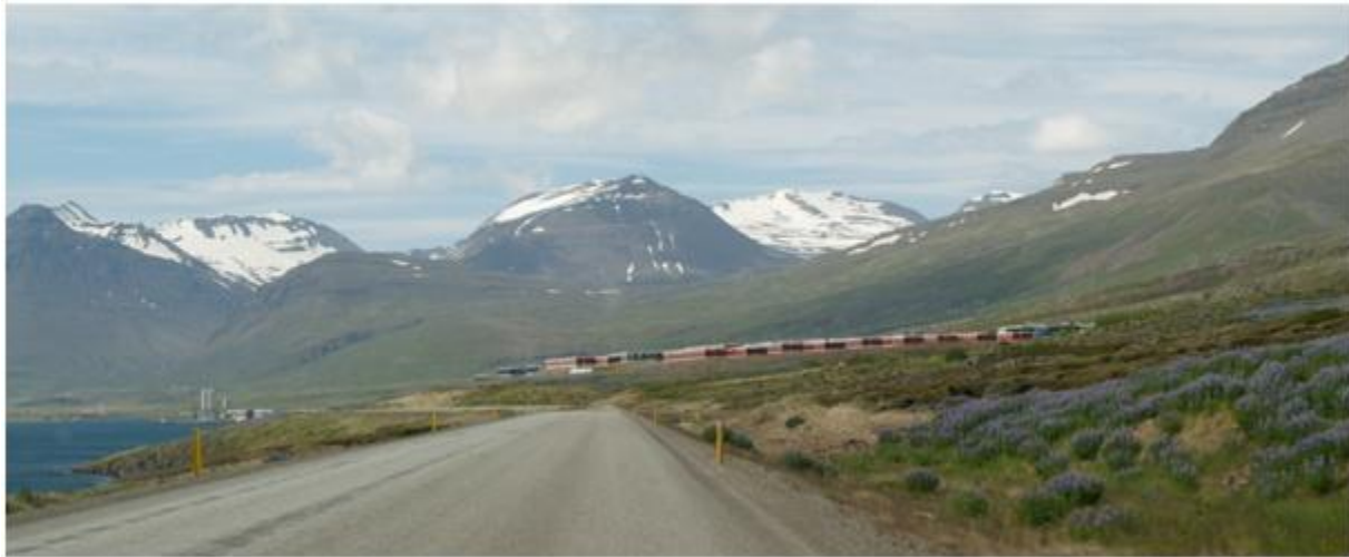
Figure 11. Workers' camp in Reyðarfjörður and the village in the distance (left) (Photo: Hjalti Jóhannesson)
