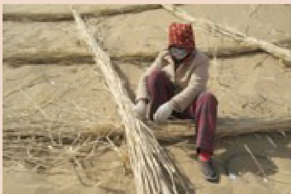
Initial stabilization of sand dunes using checkerboards
