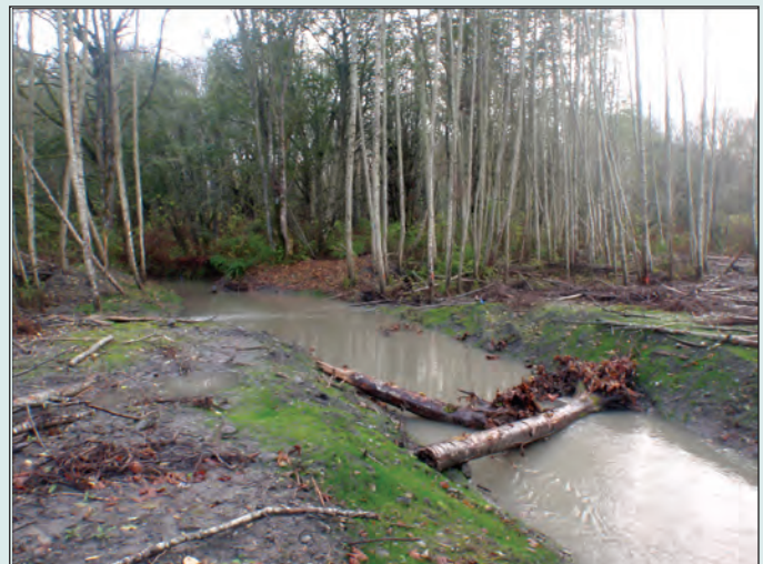
Figure S3.1.2. Newly activated flood plain overflow channel during the first winter following removal of a 1,500 foot flood plain dike on the Elwha River, Washington, 2009.
