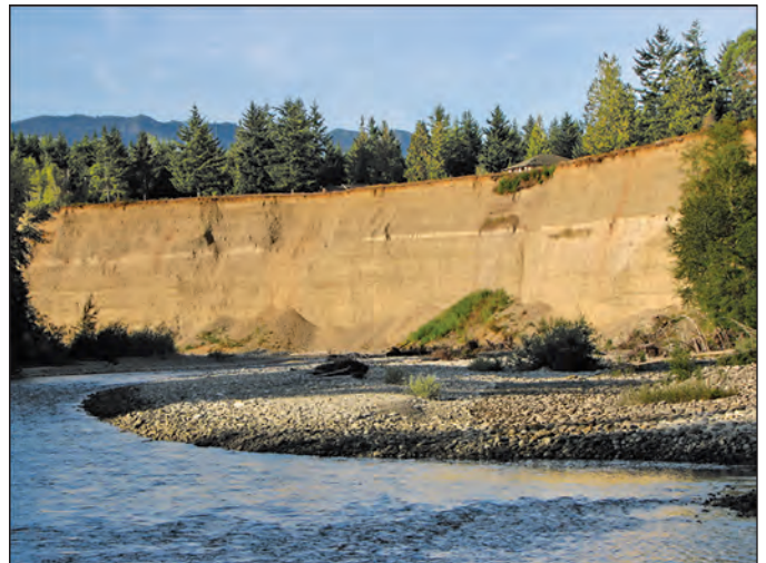
Figure 3.12. Large bluff immediately upstream of the mouth of the Elwha River, Washington. This bluff has eroded substantially during the past several decades, and it may be a primary source of sediment to the lower river and littoral cell. (Photograph taken by Amy E. Draut, U.S. Geological Survey, September 8, 2008.)
