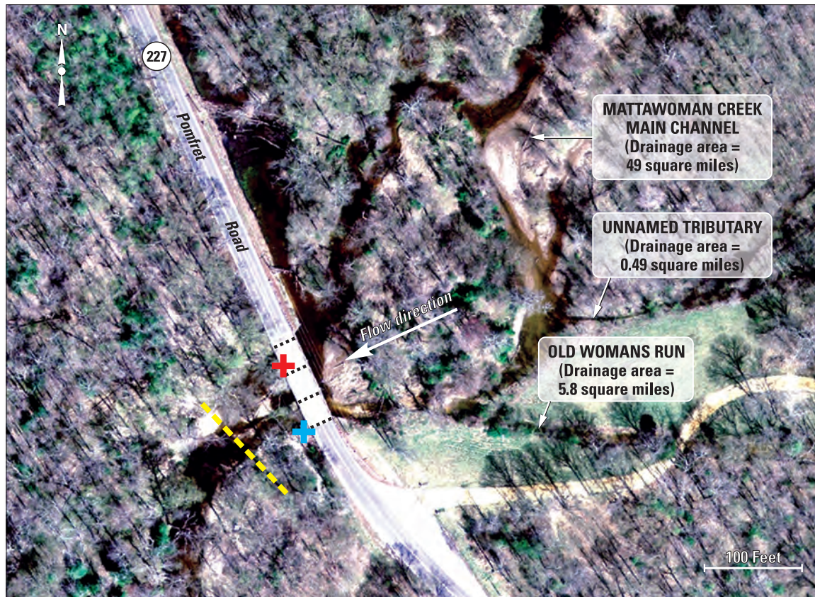
Figure 4. Aerial orthophotograph of the gage location showing location of main channel braids and the mouth of Old Womans Run relative to the location of the gage, continuous water-quality sonde, and sampler intake, 2007 (source: U.S. Geological Survey National Geospatial Program). [Blue cross indicates location of the operational sonde and auto-sampler intake; red cross indicates location of the temporary sonde deployed in 2011; yellow dashed line indicates location where equal-width-increment (EWI) samples are collected; and black dashed lines indicate positions of flow-segregating bridge supports (underside of bridge)].
