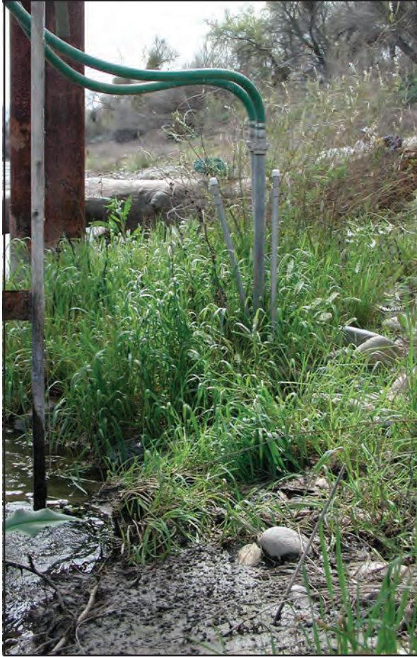
Figure 35. In-stream wells at the San Joaquin River at the Vernalis site during low-flow conditions. Photograph by Peter Dileanis, U.S. Geological Survey.
