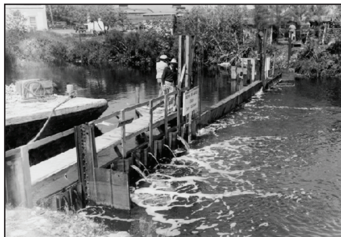
Figure 12. First water control structure on the Miami Canal installed in December 1939. This structure leaked considerably and also was opened to allow barges to pass. Photograph from the files of the U.S. Geological Survey.
