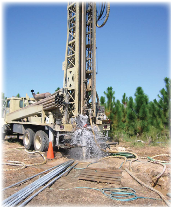
Figure 10. Installation of monitoring well CTF-228 using the mud-rotary drilling method, east of McBee and north of S.C. Highway 151 East, September 9, 2010. Water coming from the top of the borehole is return flow from advancing the drill bit and does not represent artesian conditions. The trees in the background are young longleaf pines and are characterized by a root system that can tap deep groundwater (photograph by James E. Landmeyer, U.S. Geological Survey).
