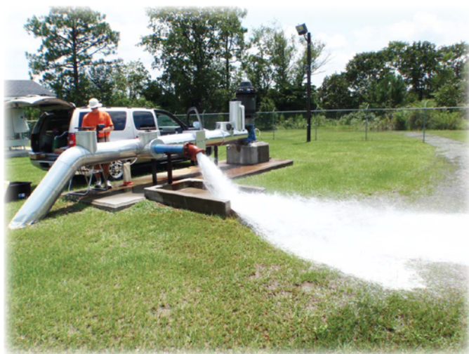
Figure 4. Public-supply Well 8 being pumped at nearly 1,000 gallons per minute prior to being sampled on August 4, 2010, for this study (photograph by Bruce G. Campbell, U.S. Geological Survey).
