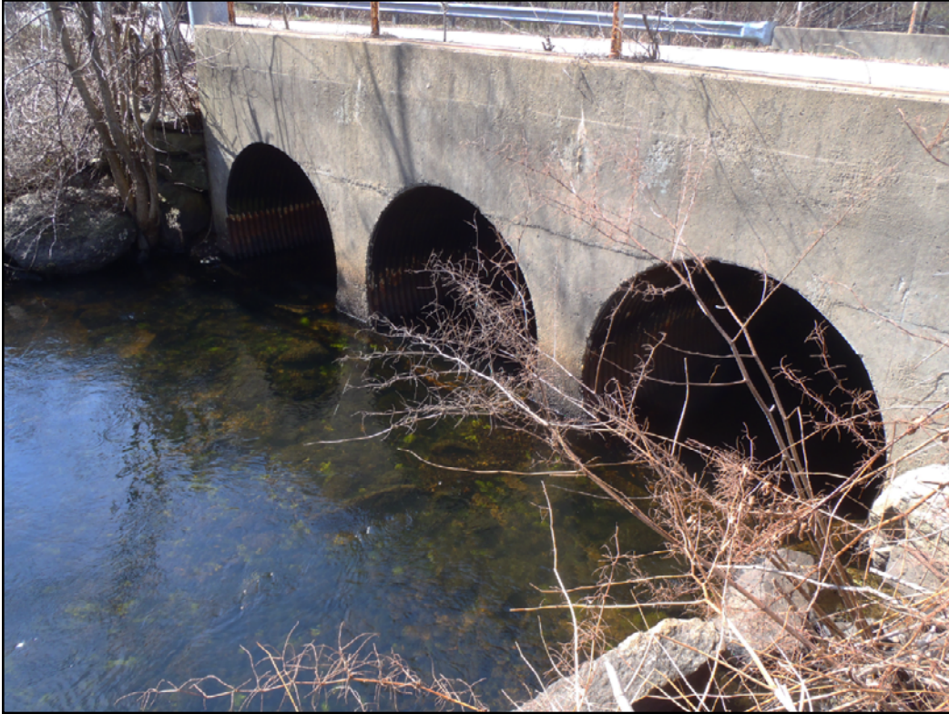
Figure 4. Downstream face of Richardson Avenue crossing Wading River in Norton, Massachusetts.
