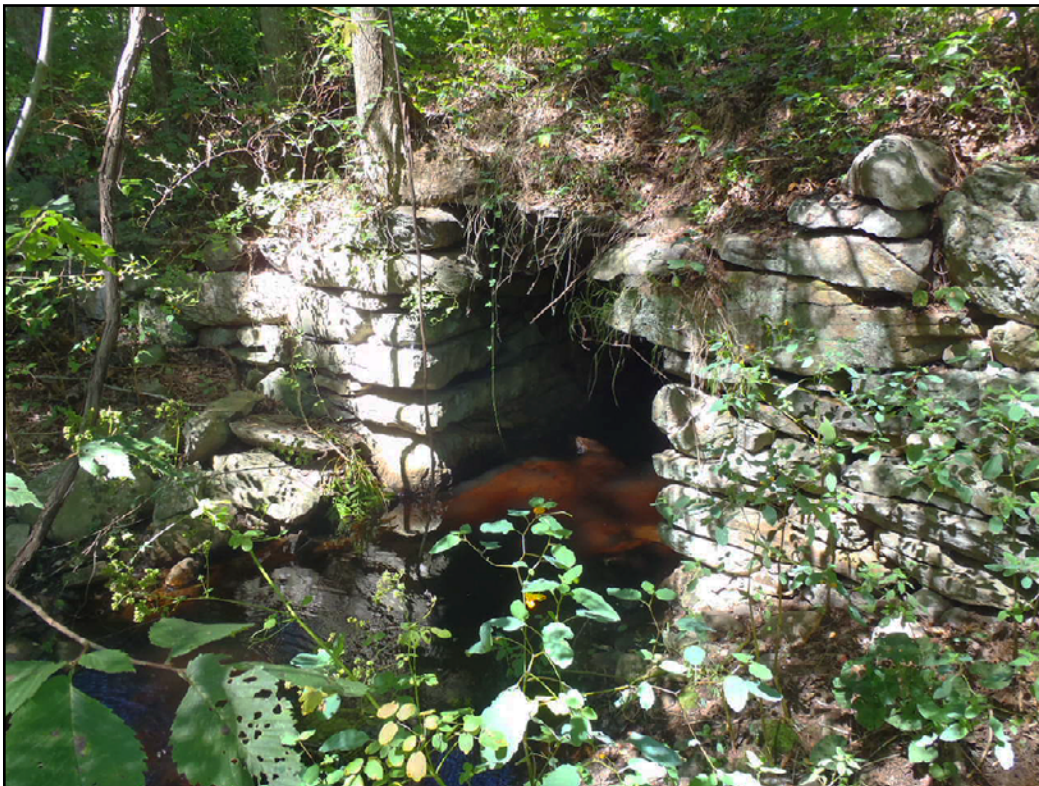
Figure 6. Downstream face of Glebe Street crossing Segreganset River in Taunton, Massachusetts.
