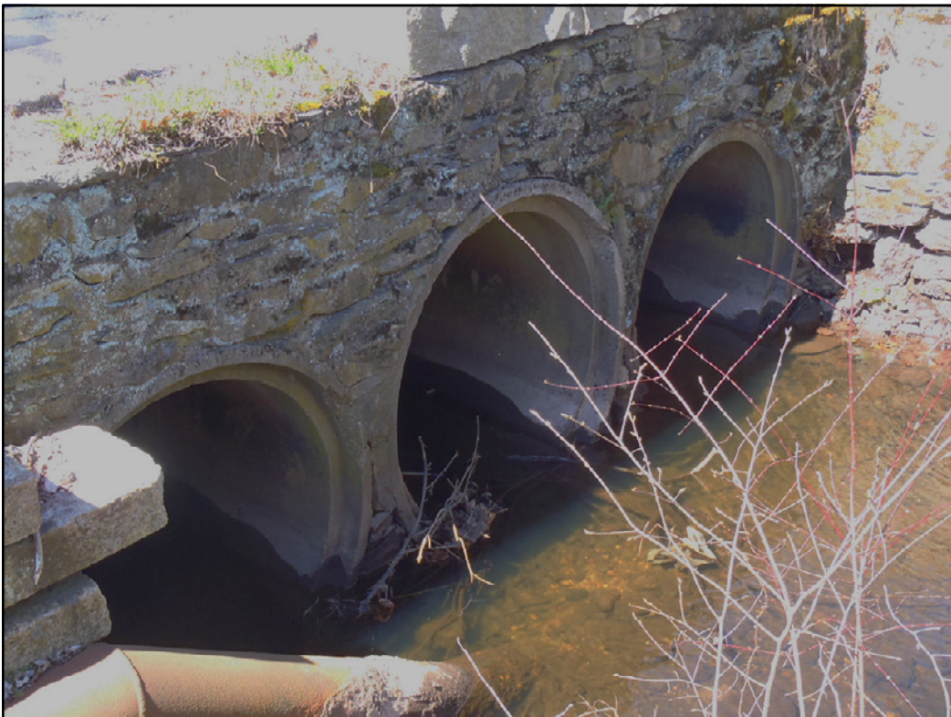
Figure 5. Upstream face of Read Street crossing Sevenmile River in Attleboro, Massachusetts.
