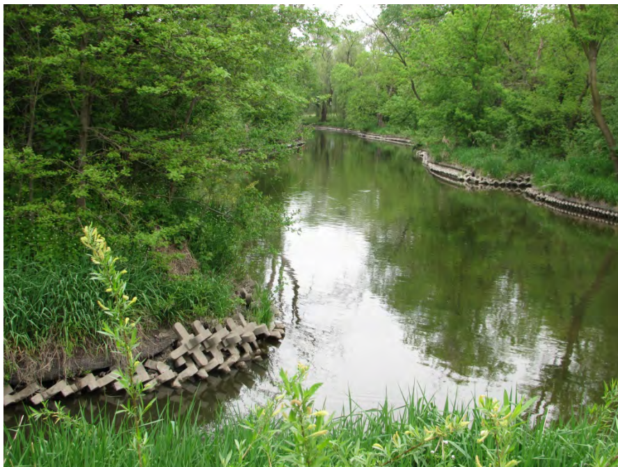
Figure 9. Photographs showing Salt Creek drainage in the study area, Elk Grove Village, Illinois, May 17, 2013. A , Near observation well TW6, looking downstream. B , Near well TW9, looking upstream.
