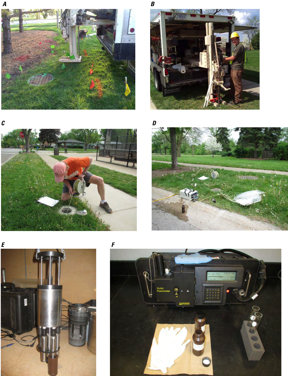
Figure 15. Field and benchtop instrumentation used in the determination of consumptive use in the study area, Elk Grove Village, Illinois. A , Direct-push system, prior to installation of observation well TW12 adjacent to a sanitary sewer line and manhole. B , Direct-push system, installation of well TW2 near the sanitary sewer lift station. C , Completed flush-mount well TW7 in a residential neighborhood. D , Completed flush-mount well TW9 in the Salt Creek floodplain. E , Fluorometer, used for in situ (field) assessment of optical brighteners. F , Fluorometer, used for benchtop assessment of optical brighteners.
