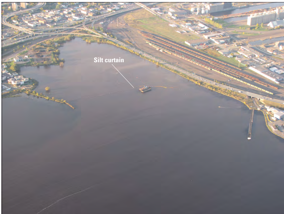
Figure 6. Silt curtain within the 21st Avenue West Channel Embayment of the Duluth-Superior Harbor, Duluth, Minnesota, on October 29, 2015 (photograph provided by U.S. Army Corps of Engineers).
