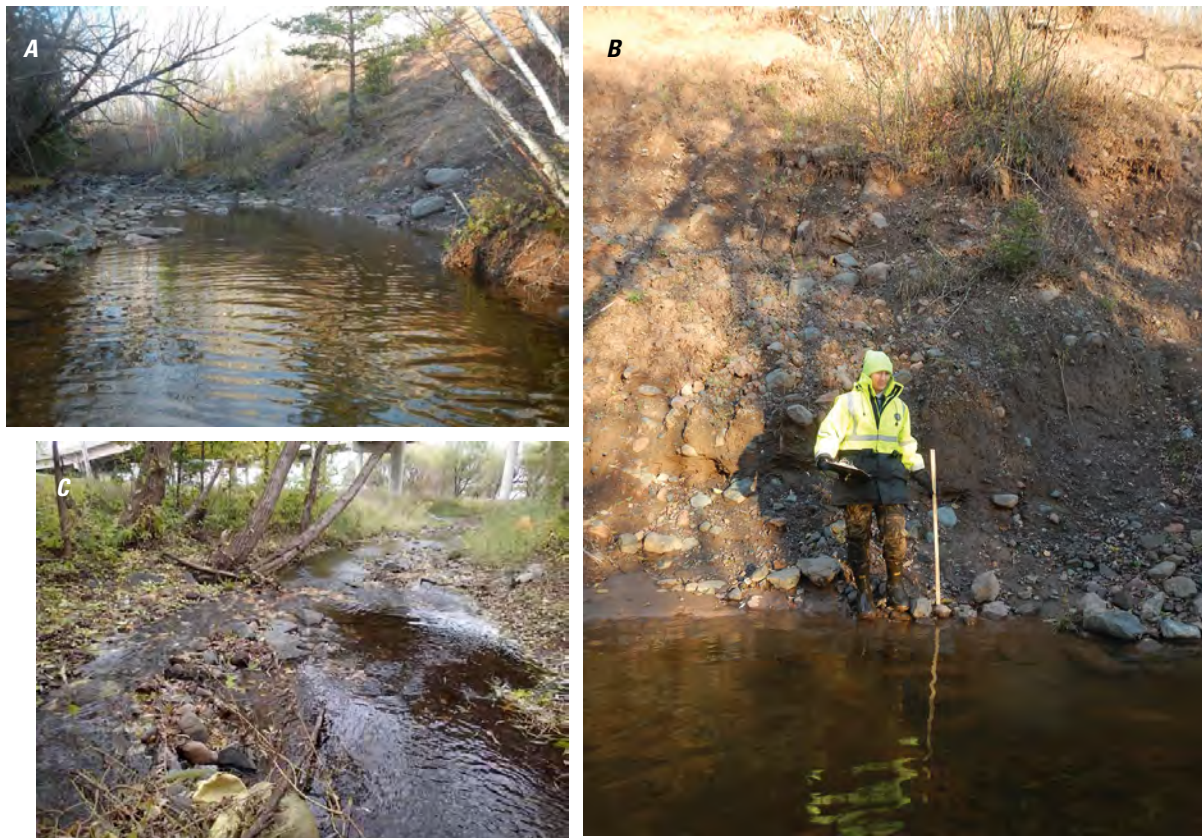
Figure 21. Comparison of erosion at selected sites in the Duluth, Minnesota, area. A and B , site 14 (Amity Creek at Occidental Road, Amity Creek Park, Number 3) that had excessive bank erosion associated with the 2012 flood. C , site 42 (Keene Creek at Bristol Street) that did not have bank erosion.
