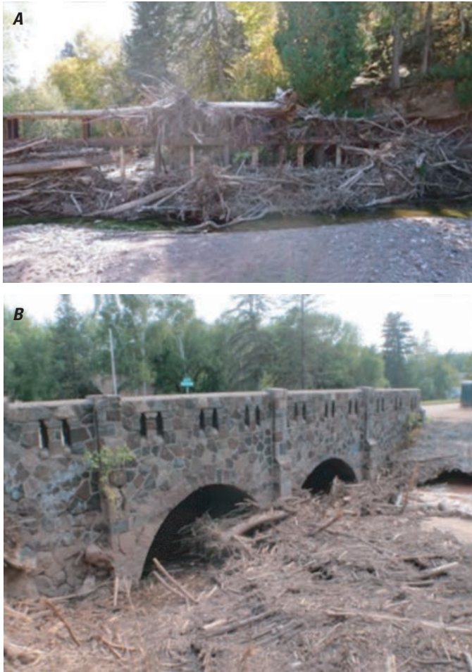
Figure 23. Large wood accumulation along Mission Creek after the 2012 flood. A , at the brush catcher. B , upstream side of bridge at State Highway 23 (Photographs by Molly Wick, Wisconsin Department of Natural Resources.)
