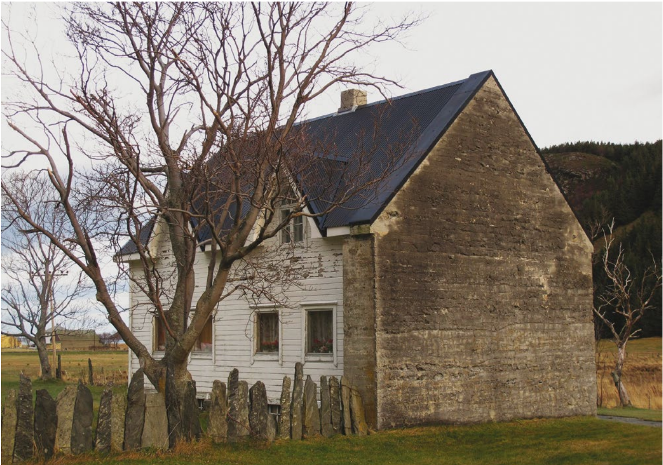
A house in Refvik (western Norway) – in this area, one side of the houses are always constructed so to withstand ice storms from a nearby lake. Photo: Torfinn Kraakennes
