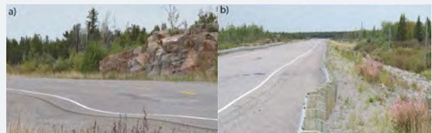
FIGURE 4: Photographs of Highway 3 indicating a) differential subsidence of the road surface and b) guardrail displacement caused by rotational down slope movement of the highway embankment side slope (Source: Stevens et al., 2012).
