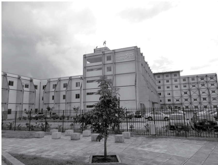
Reinforcement of the Caldas Hospital. Municipality of Manizales (Caldas, Colombia). 2011. Photography: Dora Catalina Suarez.
