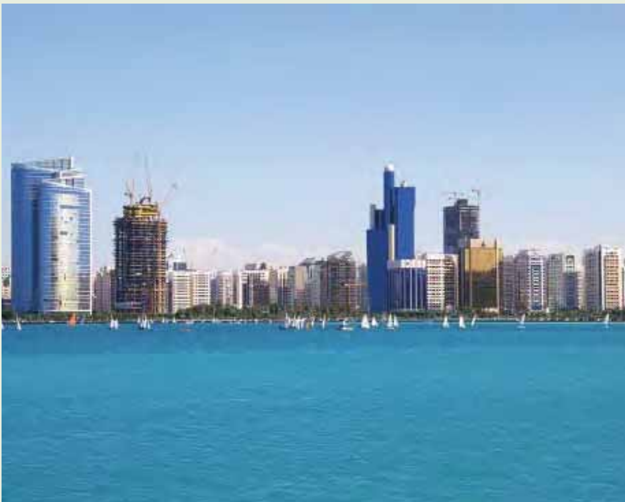
▲ On-going construction in UAE's capital, Abu Dhabi. ©Zubair Khan/Shutterstock
