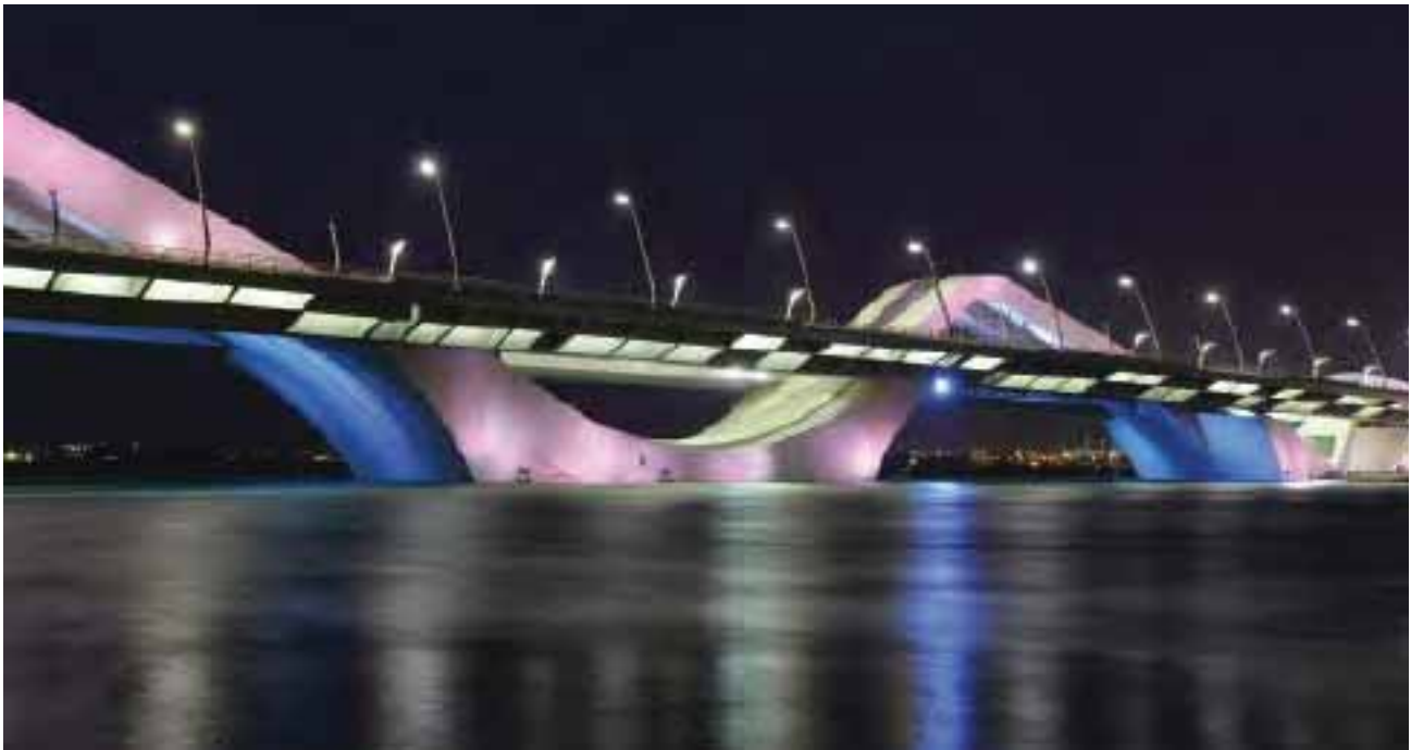
▲ Opened in November 2010, the 842 meter long Sheikh Zayed bridge in Abu Dhabi is said to be the most intricate bridge ever constructed. ©Philip Lange/iStockphoto
