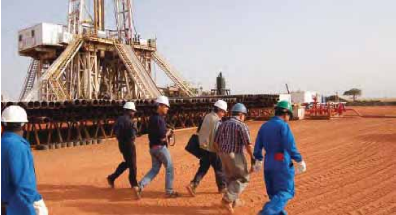
▲ Well casings lined up beneath a Heglig drilling rig in South Kordufan, Sudan. ©UNEP
