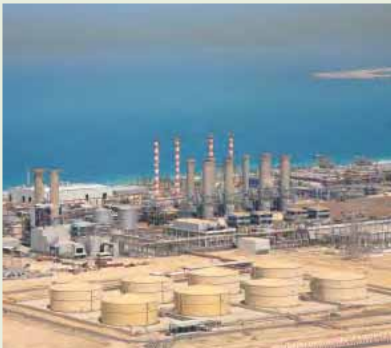
▲ Desalination plant in Dubai, UAE. ©Shao Weiwei/Shutterstock
