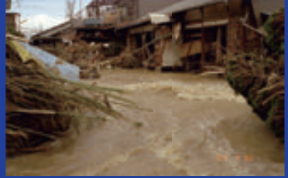
Figure 2: Damages to homes caused by sediment disaster (Yamaguchi District)
