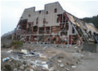
Figure 1 Tsunami damage Toni elementary school
