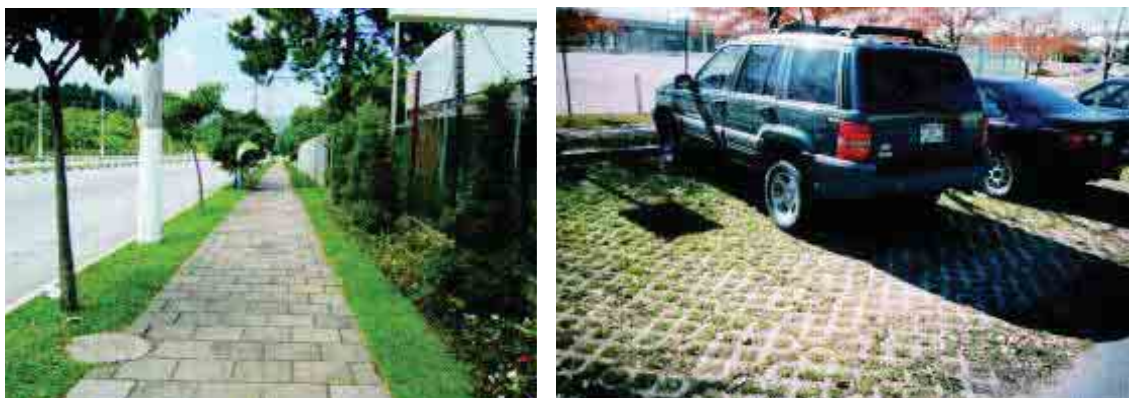
Figure 5.19: Photo (left) paths with grass alongside to increase infiltration; Photo (right) pervious paving perforated blocks for car parking.
