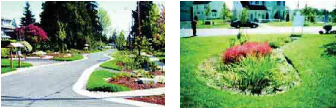
Figure 5.20: The photo (left) shows a street that allows part of the runoff to infiltrate into grass alongside (Mimicking, 2004). The photo (right) depicts an infiltration area in a flower bed (Weinstein, 2003).
