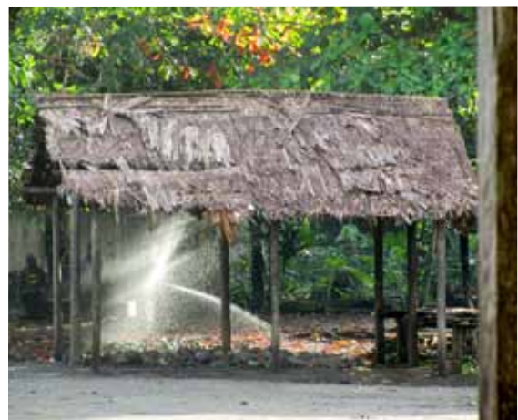
Plate 23. Water supply standpipe in need of repair
