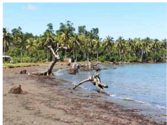
Plate 7. Mangrove removal heightened the damage by the 2007 tsunami on the coastline, and increased the susceptibility of the coastline to erosion and recession.
