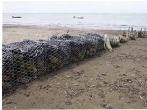
Plate 5. A local attempt to build a groyne to slow down rapid coastal erosion. This groyne made from gabion wire and rocks fell apart in less than two years. The other side of the groyne experienced rapid erosion after it was built.
