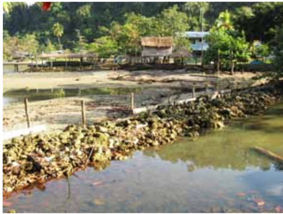
Plate 4. A seawall constructed of stones, sticks and timber. This area was previously protected by mangroves, which have since been removed, resulting in erosion, even after the construction of the seawall.
