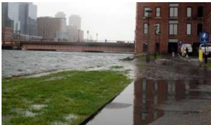
Figure 1. High tide October 29, 2012 overtops the Fort Point Channel seawall. Photo by Steve Hollander.
