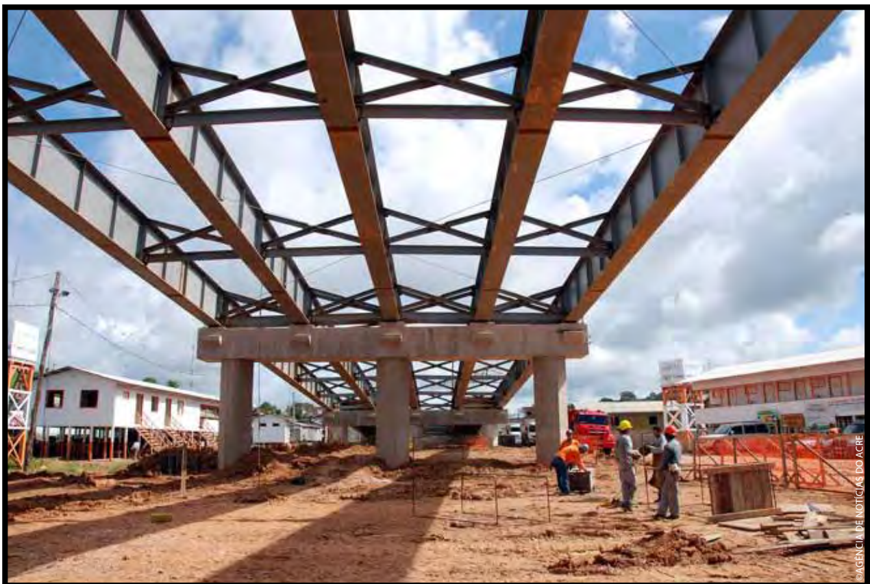
Bridge funded by the Brazilian National Development Bank: Brazil (2010).
